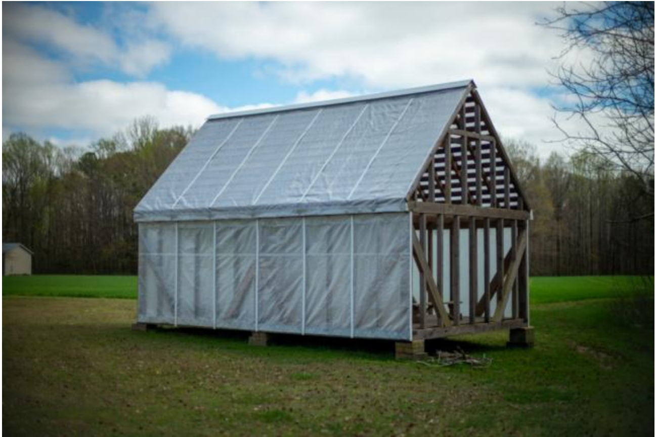
View of Remembrance Structure at Menokin (Michael Beller/Courtesy of the Menokin Foundation)
